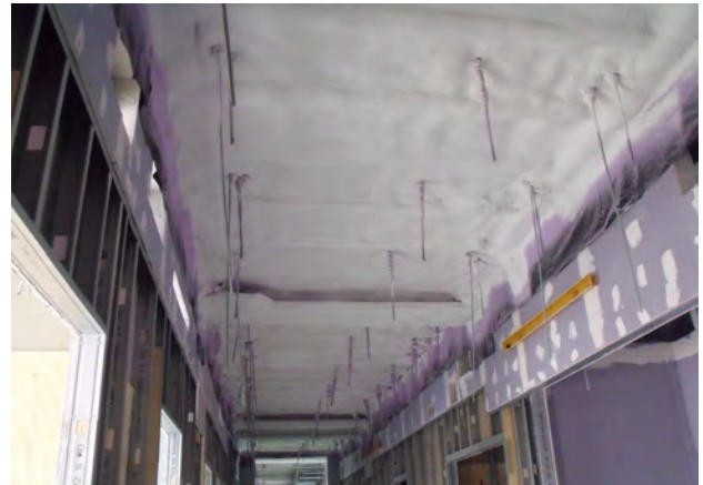
Figure 2 155mm Walltite with white intumescent coating.
