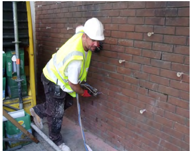
Figure 2 Martin Injecting Walltite to the lower masonry cavity
