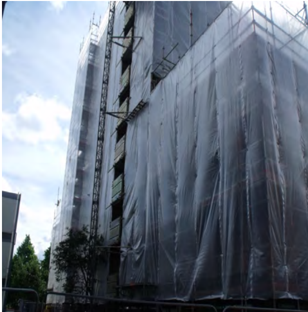
Figure 1 The scaffolded exterior of the Main Building
