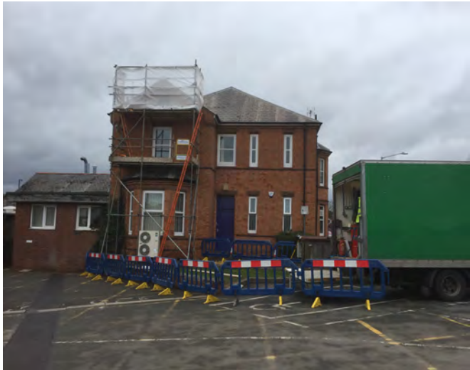
Figure 1 The scaffolded exterior of the Management Building
